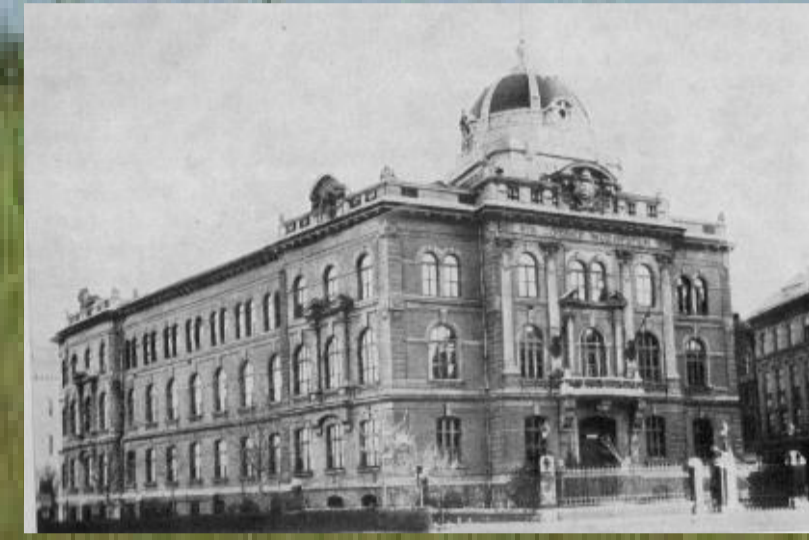
The chemical building of the Technical University
